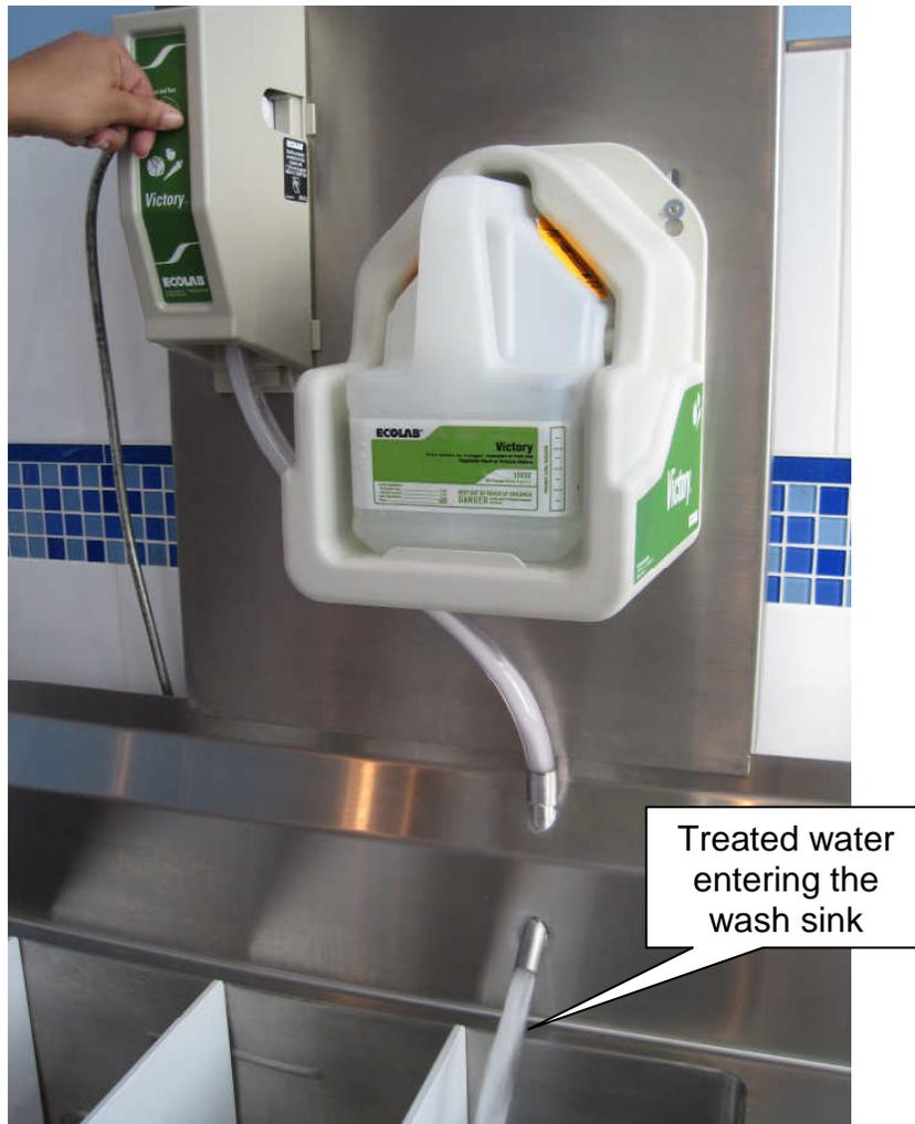
Fill the sink until the solution has reached the water level mark in the sink.
