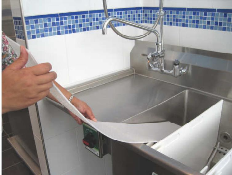
Begin bending the flow guide to the shape of the front rib set, and allow the notches of the flow guide to engage the hooks of the rear rib set.
